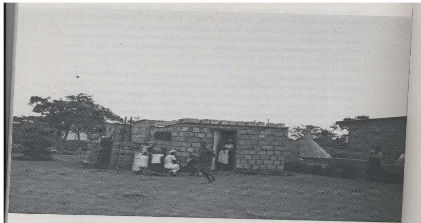
Figure 6: A household relaxing in front of their ‘house.’ This house was constructed without any regard for building regulations
