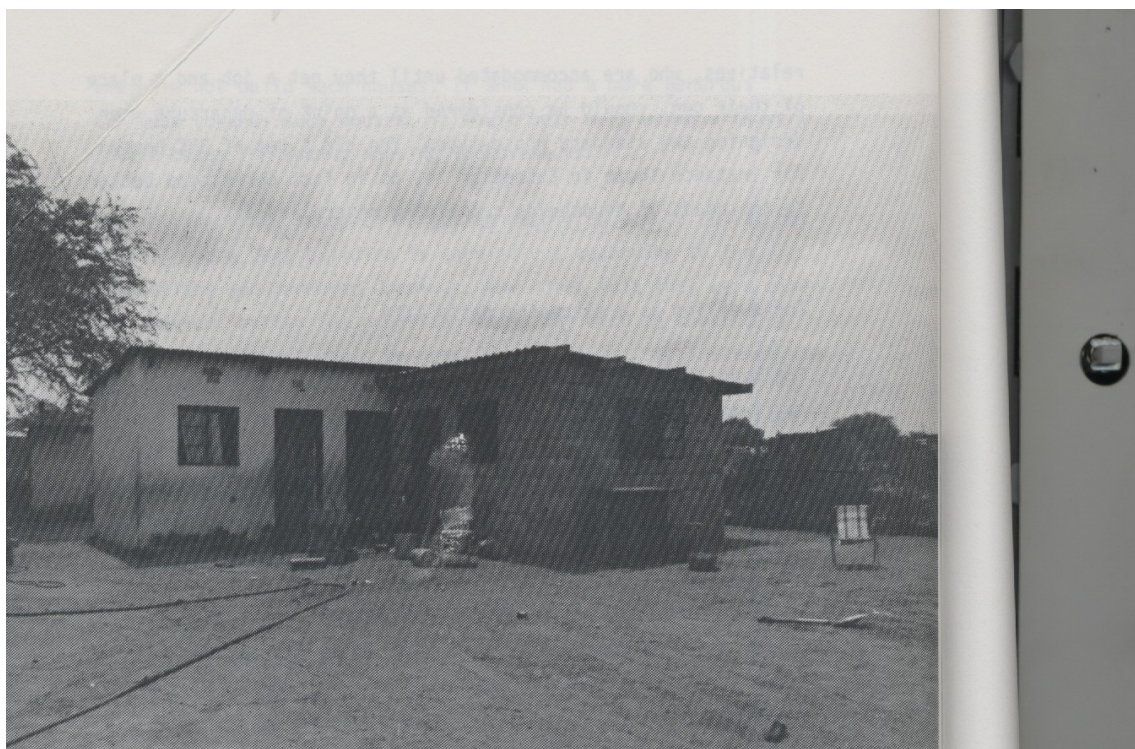
Figure 7: Incremental extension of a SHHA house
